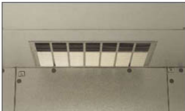
The PRS-2 evaporator grille mounts flush in a standard 4" thick ceiling panel allowing maximum storage space.
